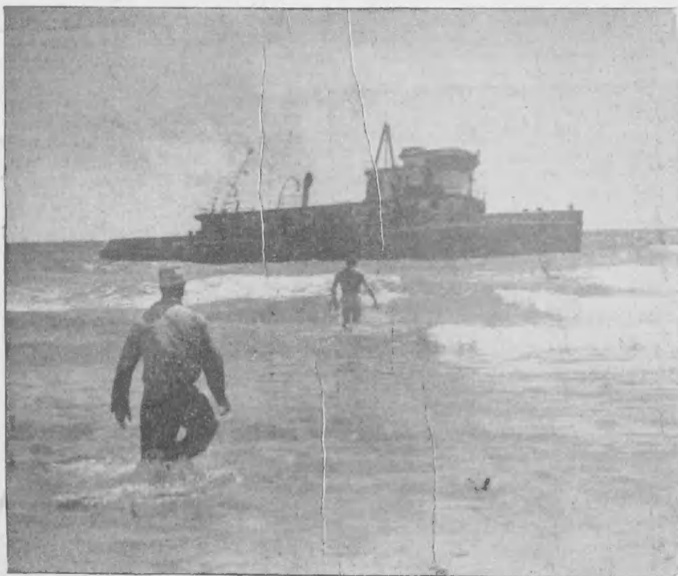
The Captain Rodger, a constant reminder of the ocean's power, may soon be demolished by men of the Shipyard. The Rodger, wrecked when it attempted to aid a foundering tanker, is now wedged on a reef on the north-east coast of Aruba. At present the superstructure is being removed (note that the stack is gone), although the job is made difficult by the heavy surf. Here, Welding Foreman Verl Clark (center) swims out to the Captain Rodger to complete the job of cutting the superstructure away. Lines for the torches were stretched from shore to ship. Joseph Joseph, foreground, runs into the surf to grab a line washed sideways by the waves.
